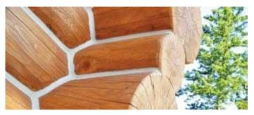
Chinking or caulking must be able to move when the wood moves.
