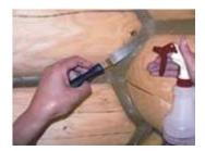
8. All joints should be tooled by spraying a small amount of water onto the chinking and smooth to the desired finish. Do not saturate the surface with water. If it begins to run you have applied too much. Always trowel in such a way as to form a good seal to the wood. Maintain a depth a little more than 1/4", as the material will shrink slightly when cured.
